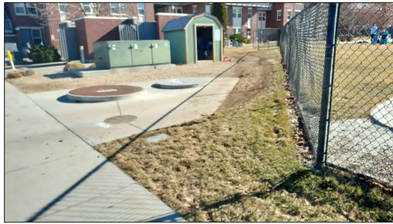
Existing Wet Well
