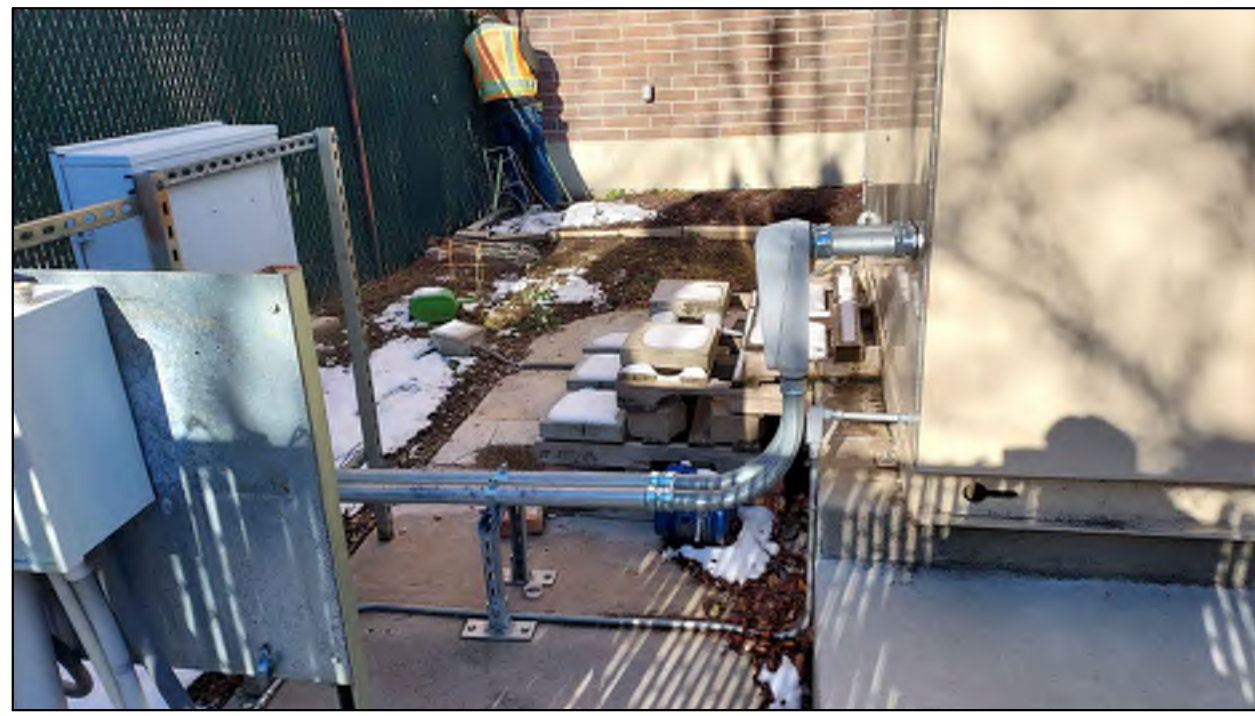
Existing Pump Station
