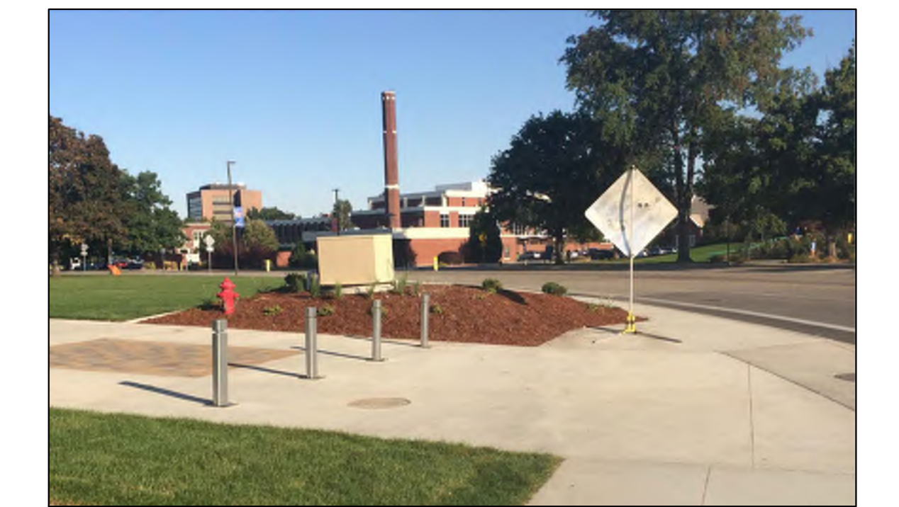
Honors College Pumpstation
