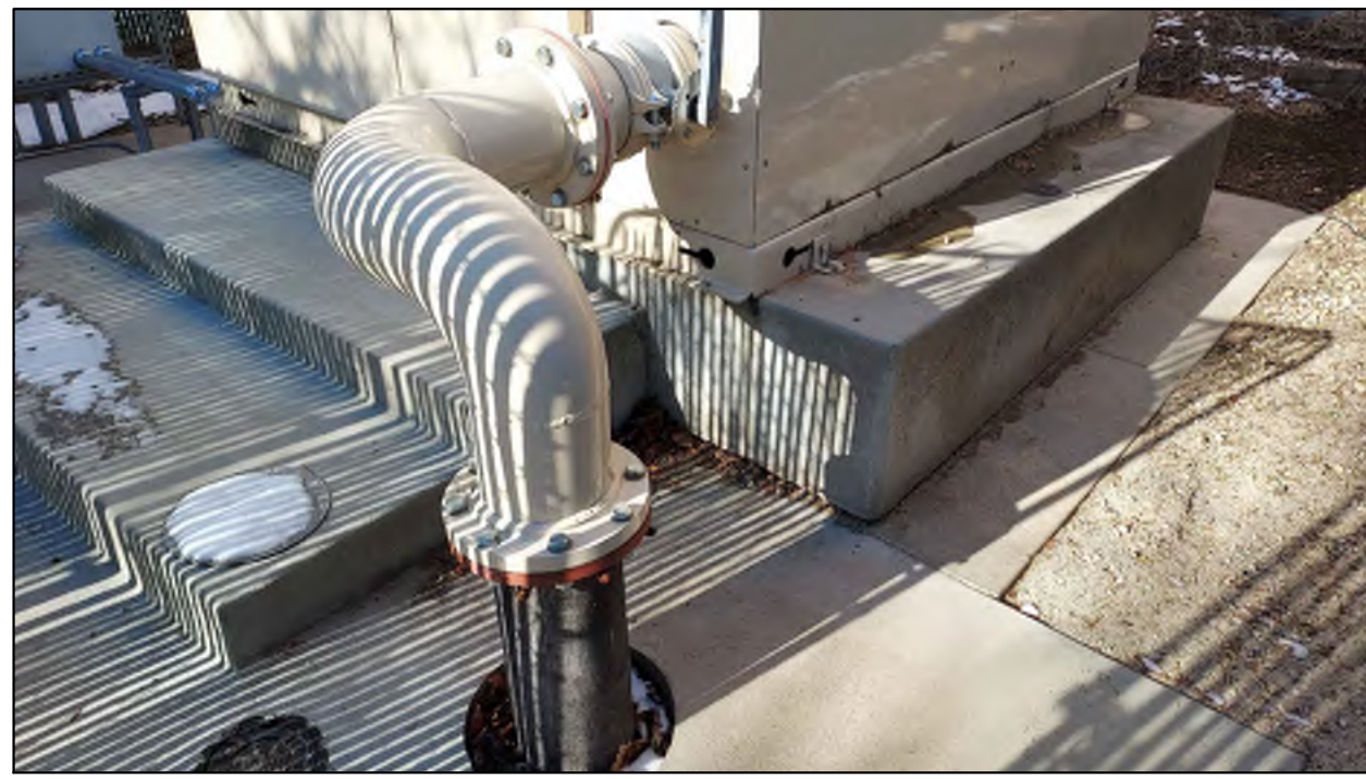
Existing Pump Station
