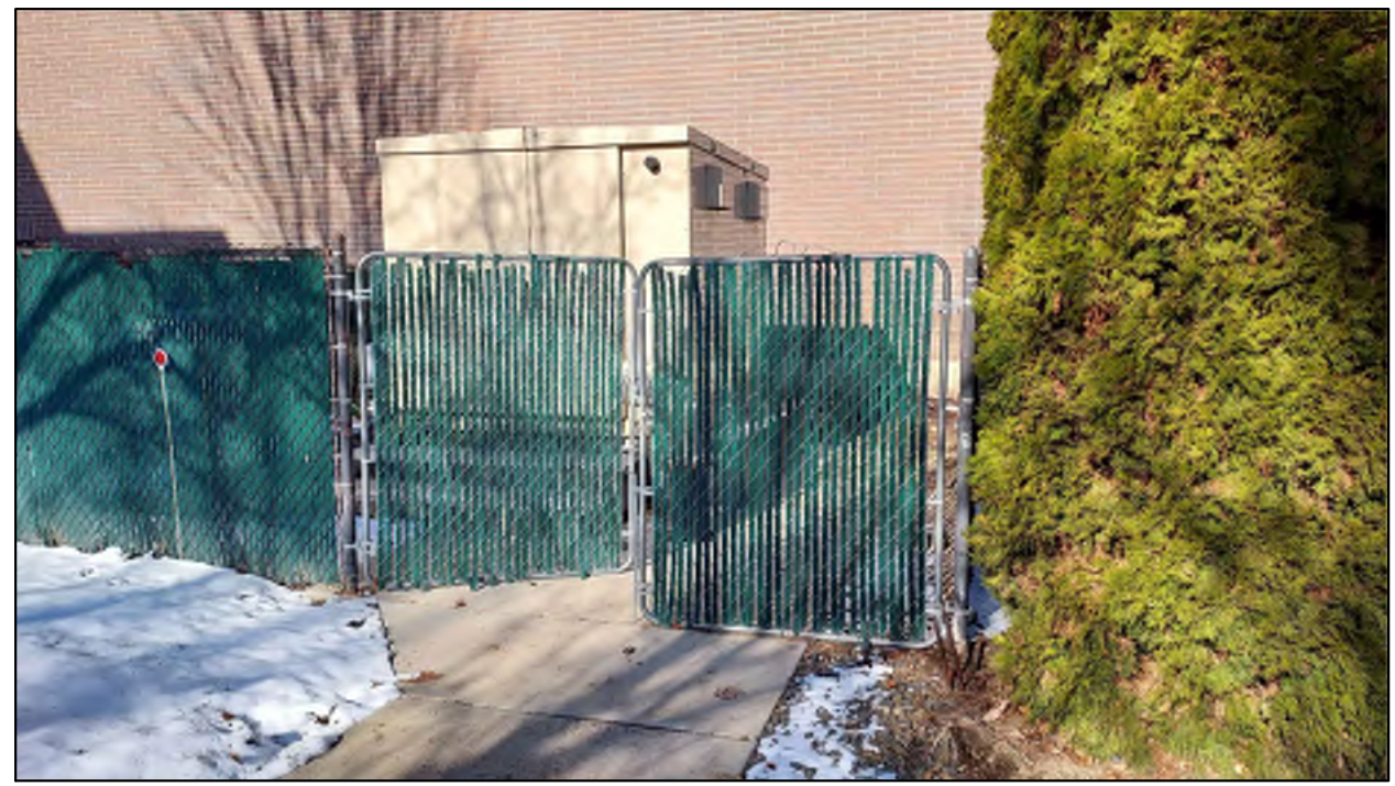
Existing Pump Station
